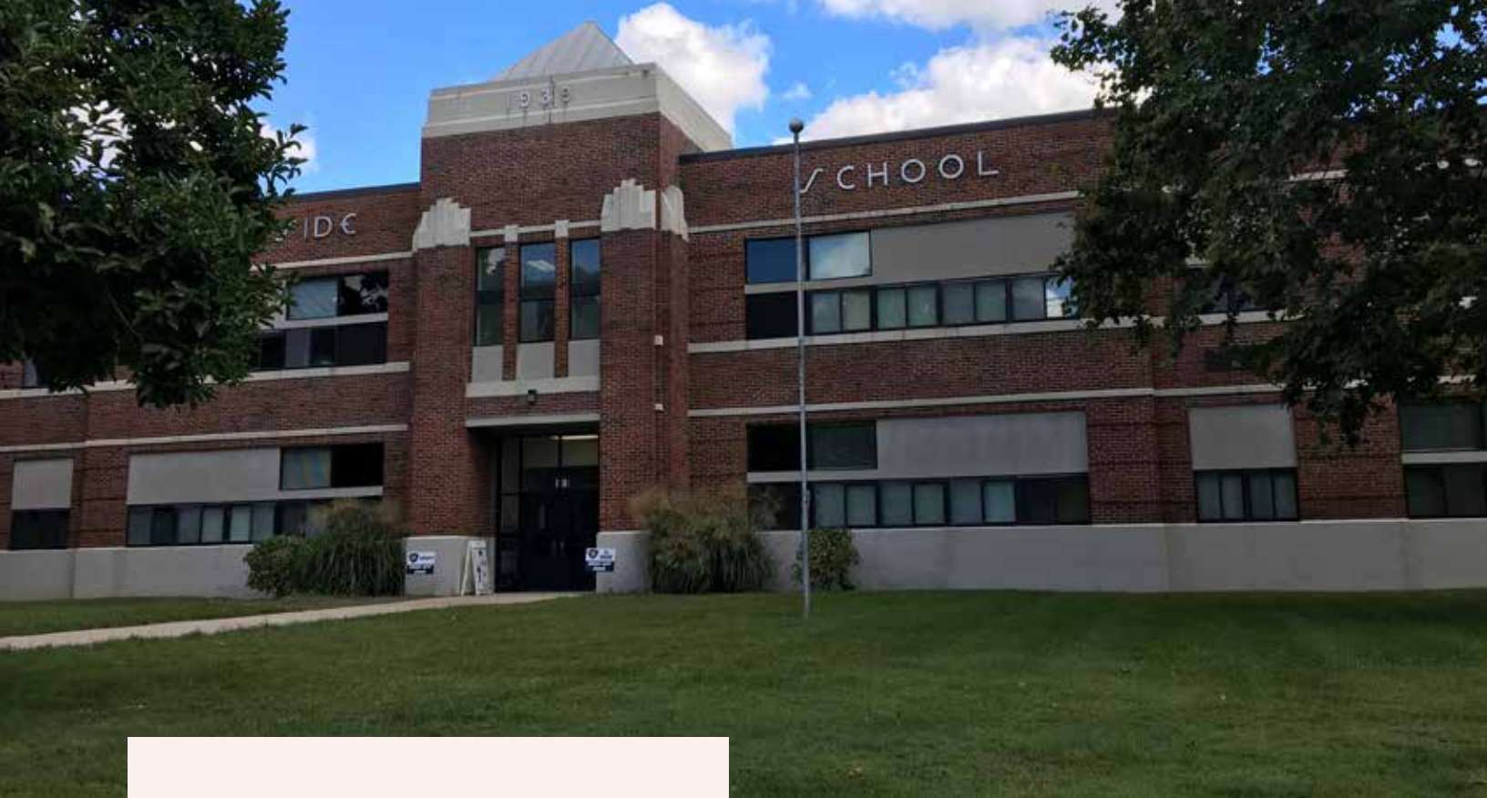
FIGURE 4-7. EASTSIDE ELEMENTARY SCHOOL
