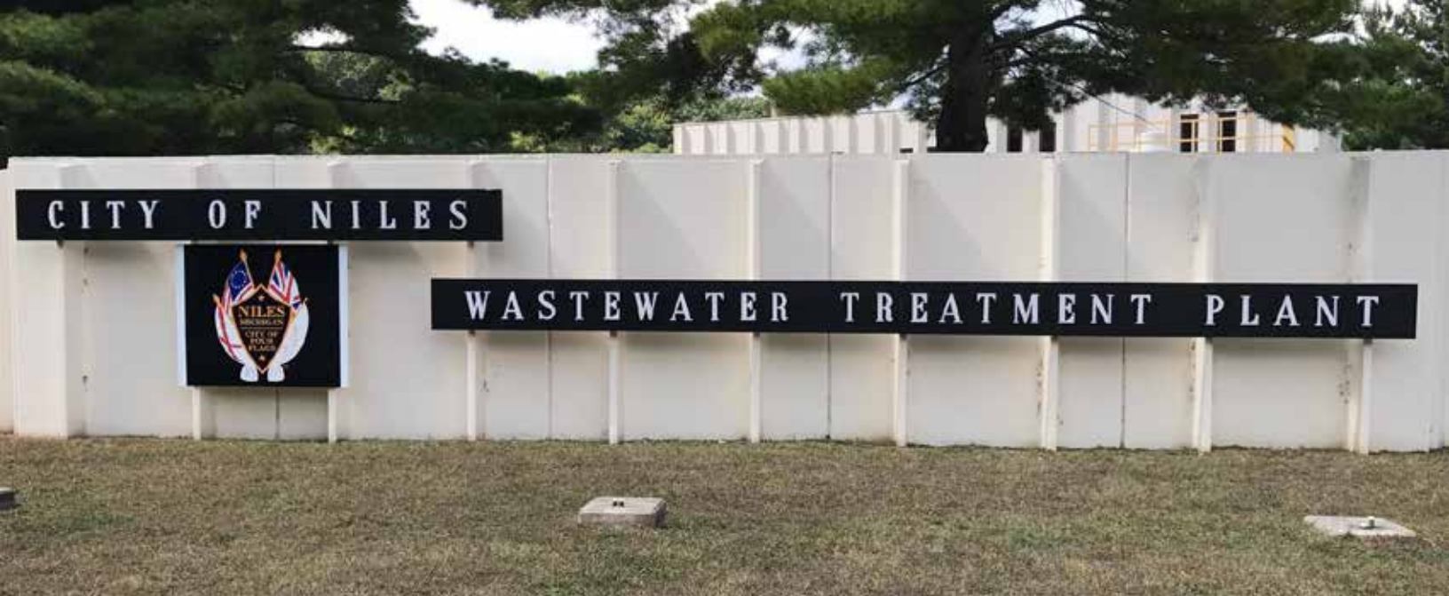
FIGURE 8-2. WASTEWATER TREATMENT PLANT
