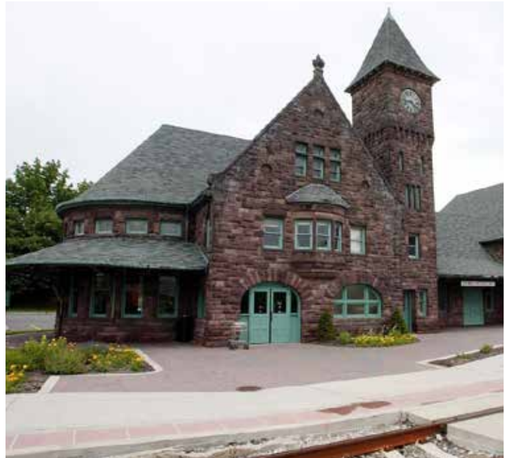
FIGURE 9-5. HISTORIC NILES AMTRAK STATION
