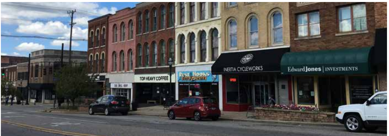
FIGURE 5-8. STREET VIEW OF THE DOWNTOWN HISTORIC DISTRICT
