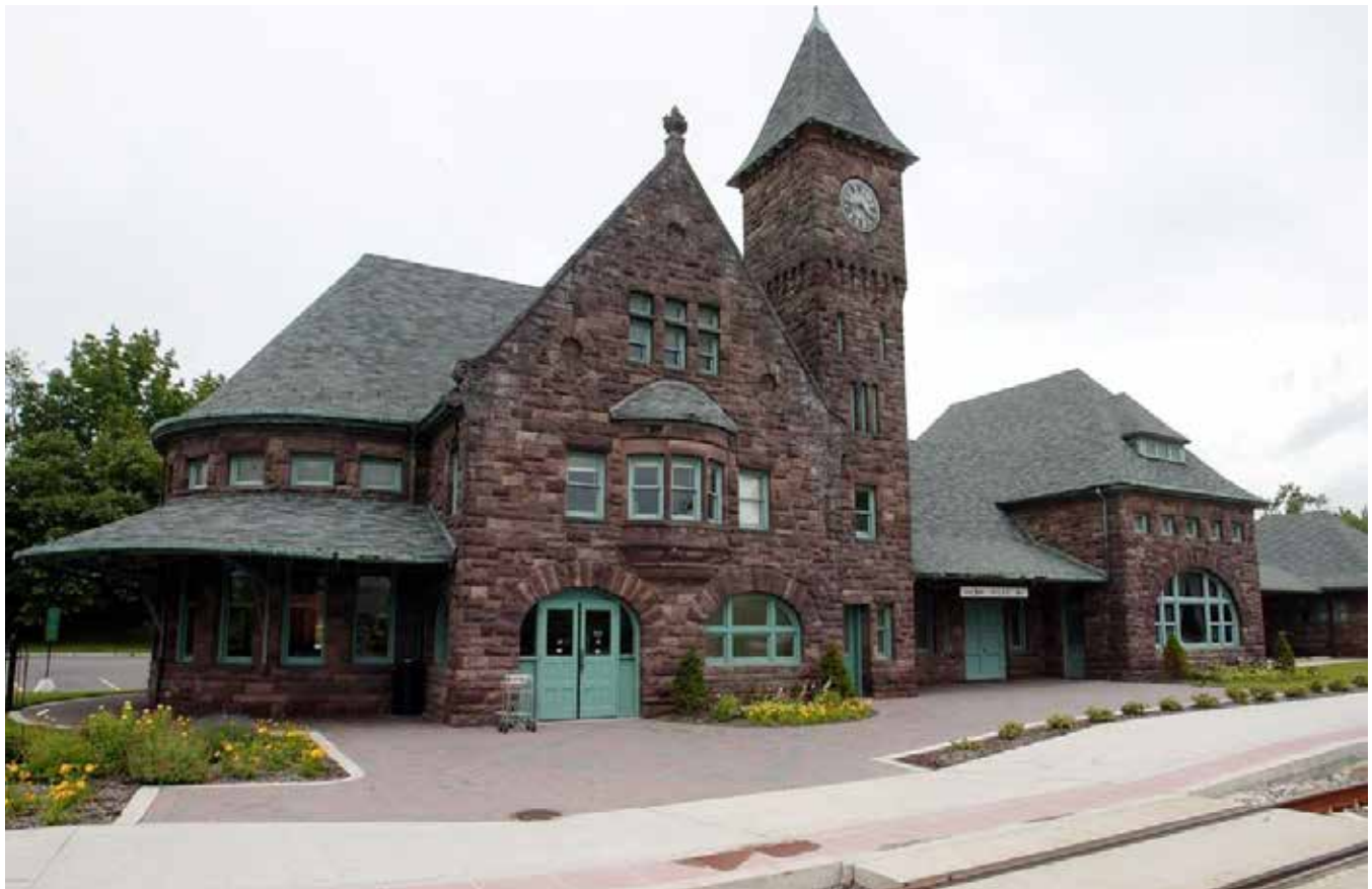
FIGURE 2-4. NILES TRAIN STATION
